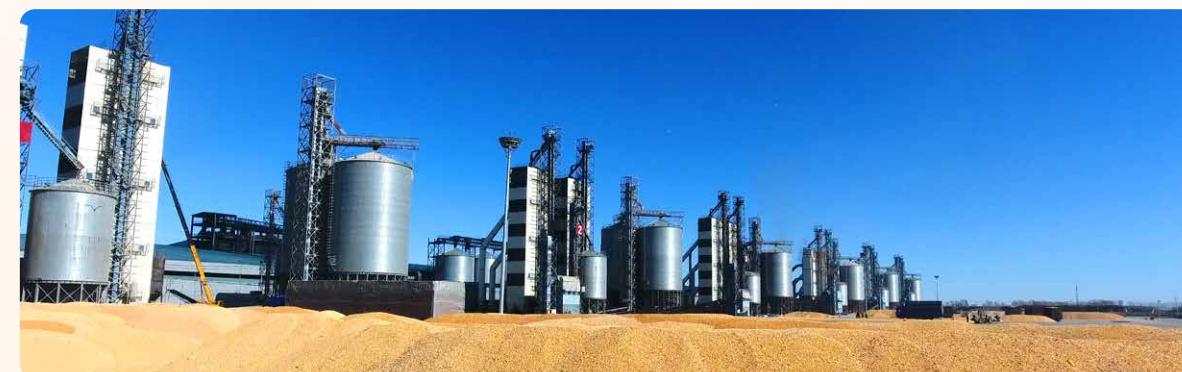
XMXYG A. G. R. I. has built seven modernized grain storage and logistics centers in key grain-producing areas
